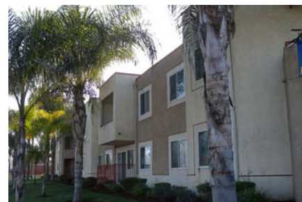
Use of bay windows, variable roof height, and facade detailing.
