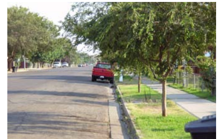
Typical streets are two-lane local streets with parking on both sides, planter strips, and a consistent row of street trees.
