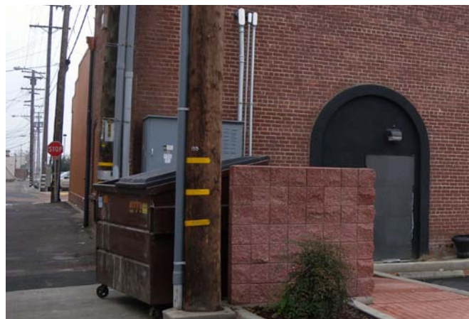
Utilities accessible from the rear alley on the side facade.
