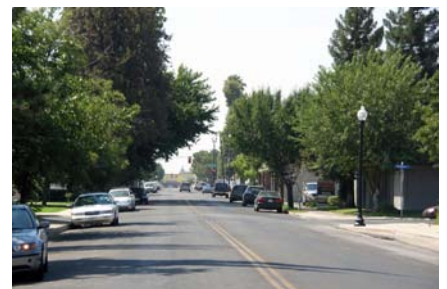
Typical streets are two-lane local streets with parking on both sides, planter strips, and a consistent row of street trees.
